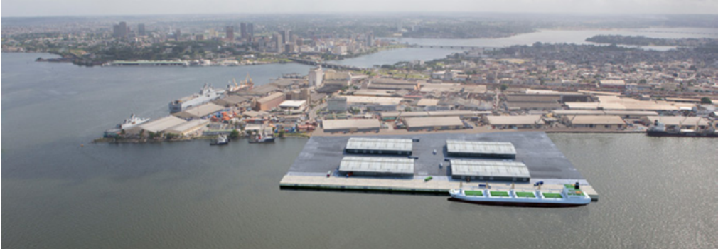
Photo : PAA / Creation of a cereal terminal (Start of works January 2020) – After works
